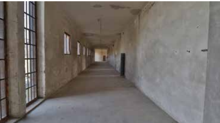
Interior view of the cell corridor, 2025 (0393 ©Peer Wittig)
